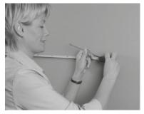
**Step 5** To install the next wallband, measure and mark out a suitable distance between the two wallband.
