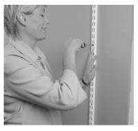
**Step 3** Drill holes and fasten the remaining screws.
