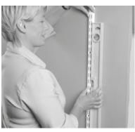
**Step 2** Check with a level that the wallband is hanging in vertical position.
