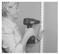
**Step 1** Position one wallband where you want it on the wall. Mark the position of the second screw hole from the top of the wallband.
